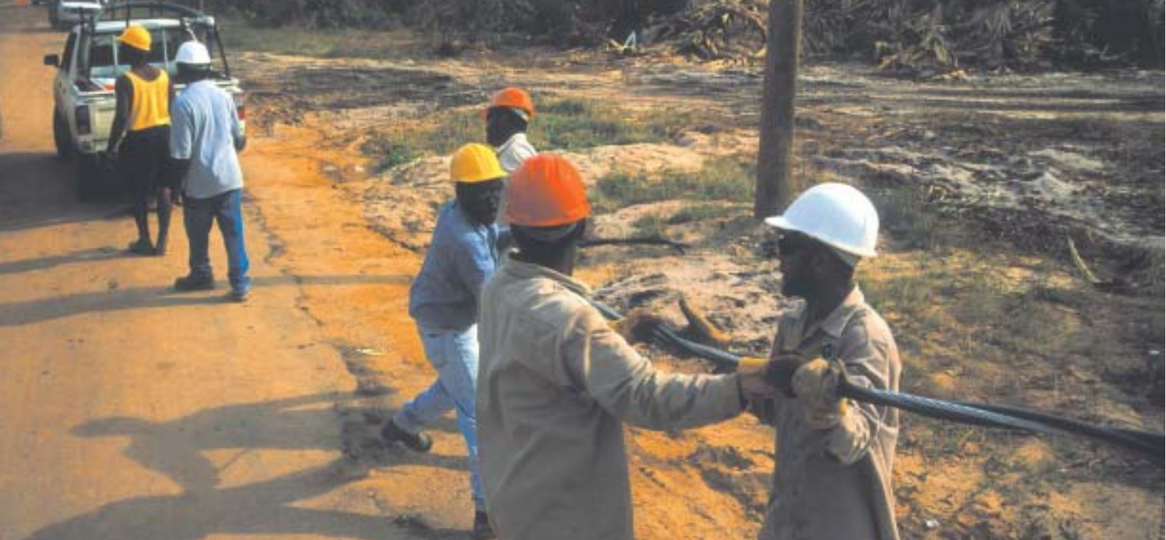
Belize Electricity employees restore service to customers affected by Hurricane Iris.
